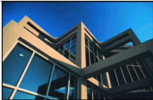
The exterior of Shaw's newest manufacturing plant in Cartersville, GA exclusively for tile, including the environmentally guaranteed EcoSolution Q and EcoWorx products.
